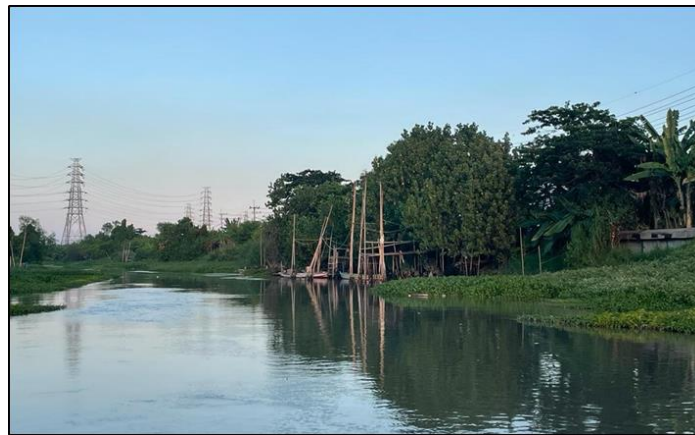
Figure 2. Construction of bamboo pier on Wonorejo River
